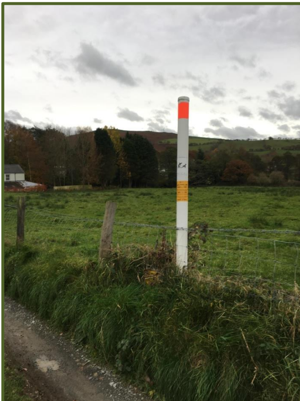
Plate 17 Gas main marker on northern site boundary .
