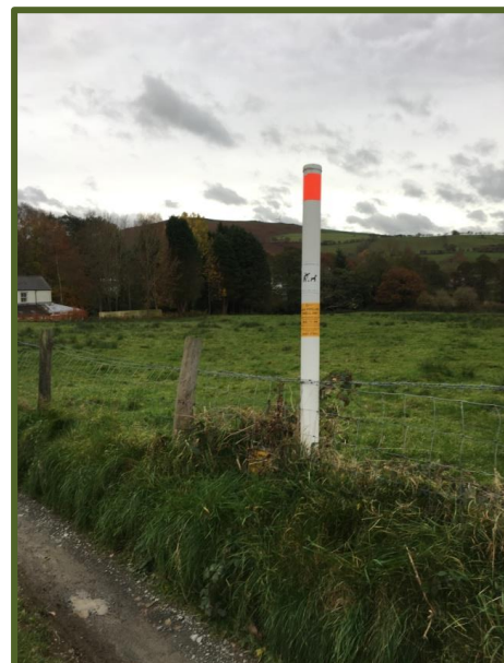
Plate 9 Gas main marker at the northern end of the site
