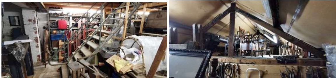
Bath Street access to loft and loft space.
